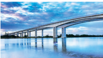
Monitor infrastructural deterioration in bridges
